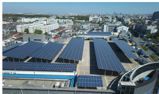
扬州印象汇光伏车棚
